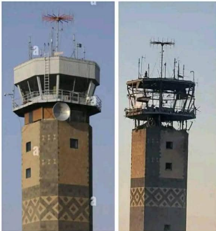
Fig. 2: Sana'a Control Tower showing the level of devastation
